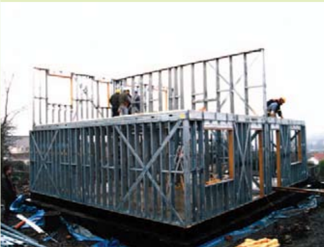
Figure 2 · Typical lightweight steel frame construction
