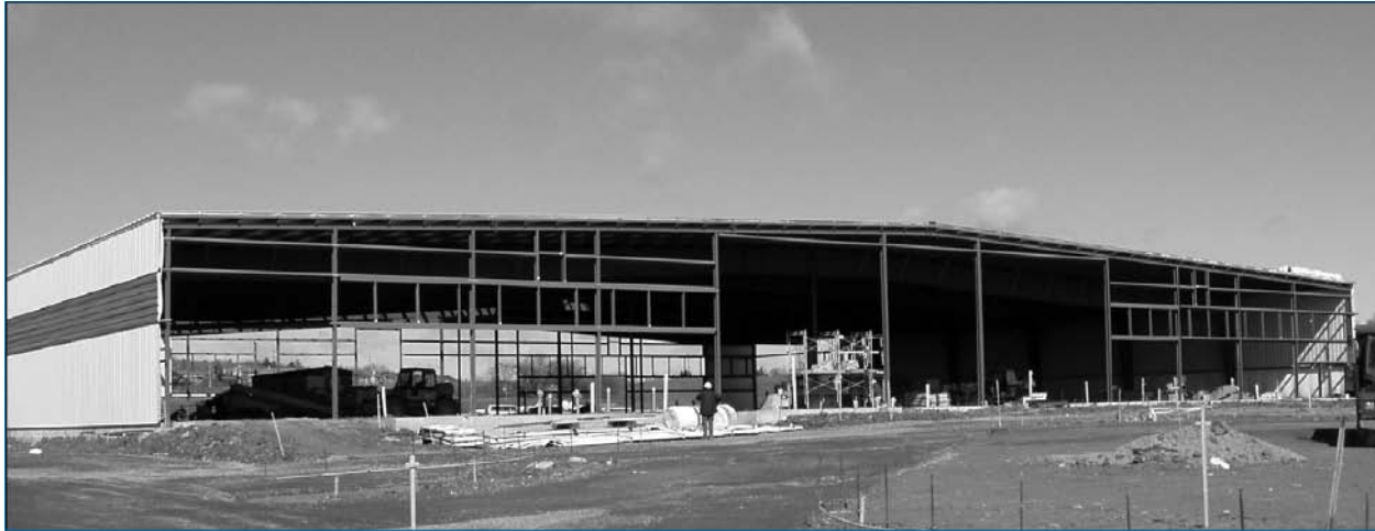
Figure 2: Typical sloped roof building site
