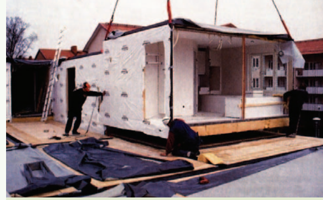
Figure 2 • Prefabrication can reduce impact of work on site
