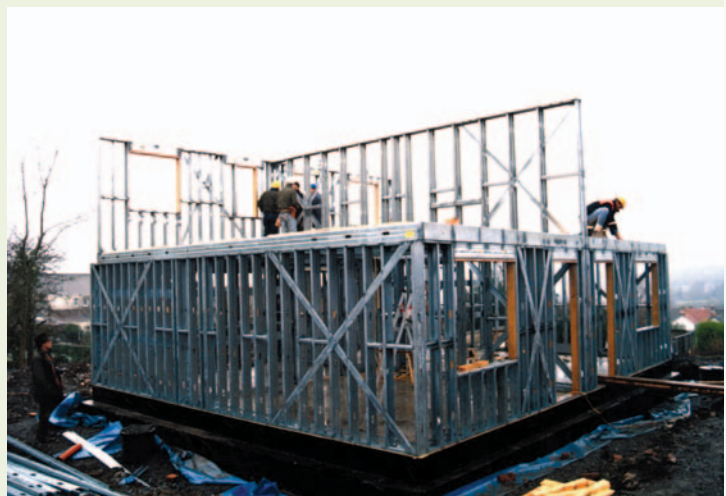
Figure 3 • Typical light steel frame construction
