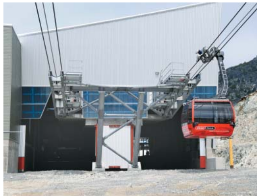
Views of the gondola station with Galvalume Plus cladding and translucent Rodeca panels, allowing views of the interior workings.
