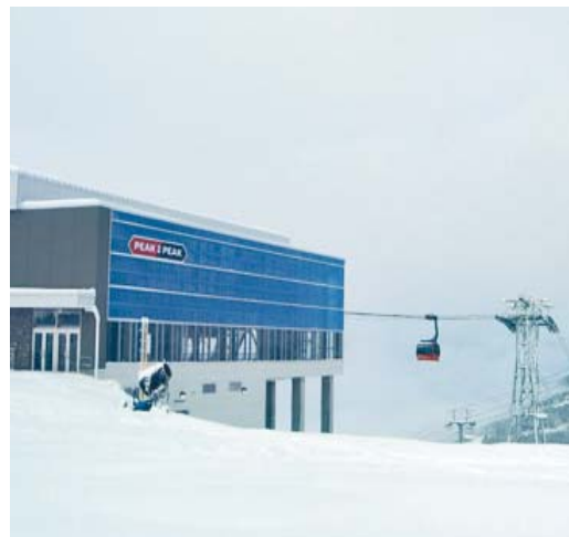
Views of the gondola station with Galvalume Plus cladding and translucent Rodeca panels, allowing views of the interior workings.
