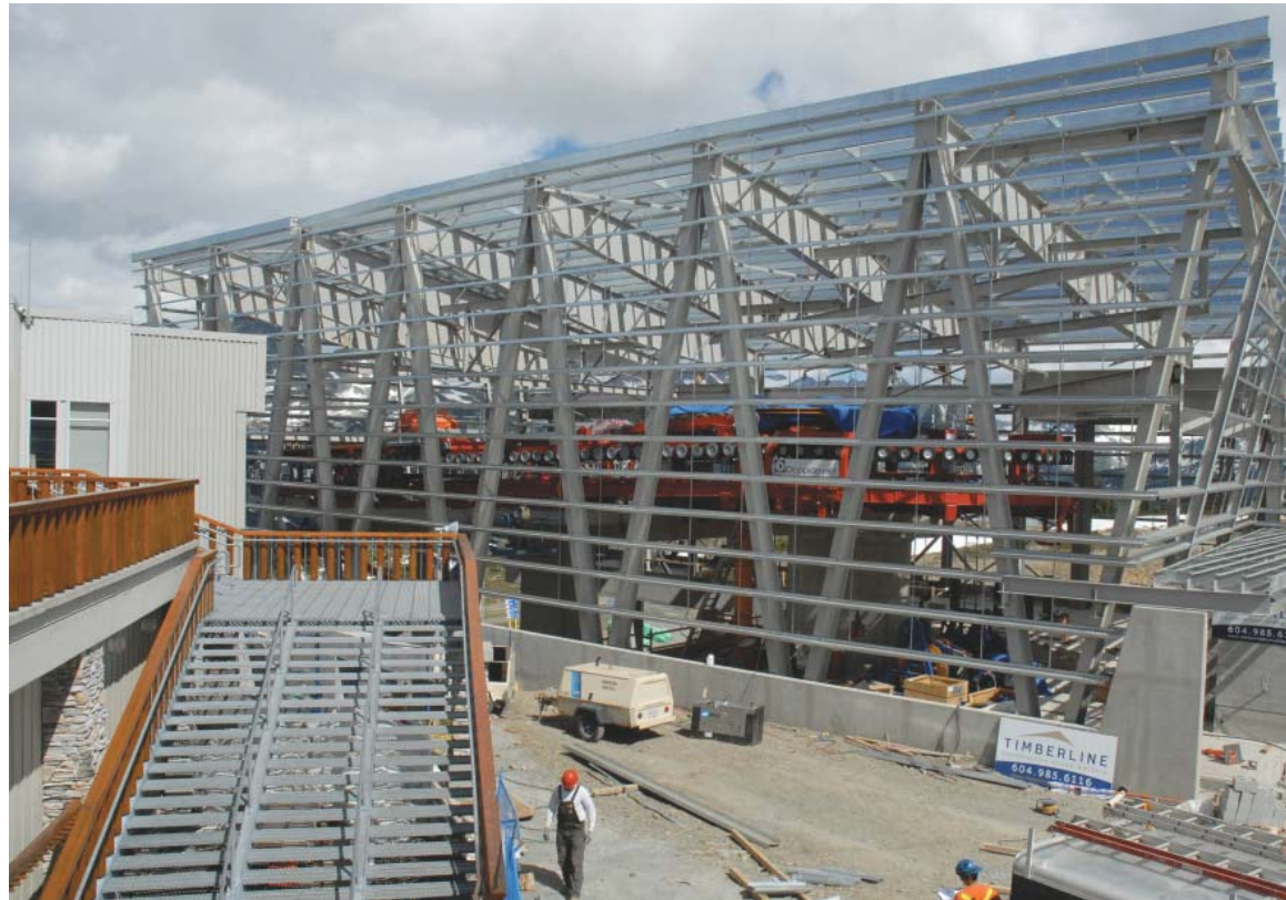
Buildings at both Whistler and Blackcomb are the FLEX-SYS® Building System from BEHLEN Industries LP. One of the advantages over other structures is that all the structural elements were manufactured in-plant and only needed assembling on site.
