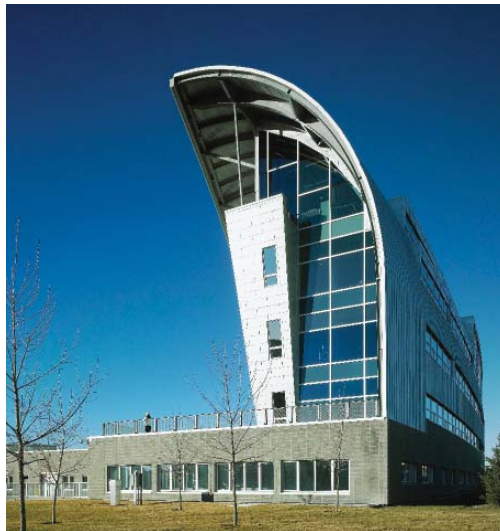
East end of building with curved roof showing glass windows on curved surface, W530 curved section soaring to a height of 20m (65.5') above floor supported by W530 sections cantilevered from the face of the building.
