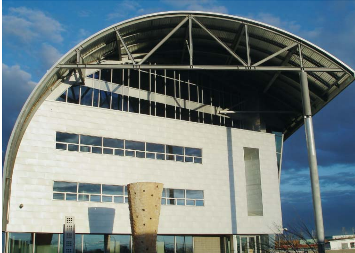
West end of the Water Centre showing maximum 4.8m (15.7') high Warren truss spanning from 15m (49') high HSS 610 column to cantilevered truss projecting from building. Also visible is the ASTM653 Grade33, Z275 (G90) galvanized steel deck and AZM165 Galvalume Plus shingle wall panels.
